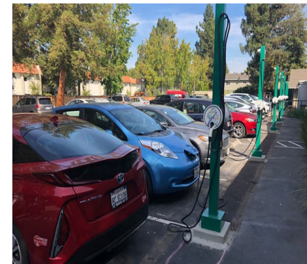
Examples of EV charging co-located with parking lot area lighting.
