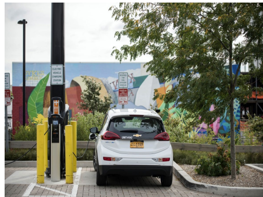
Examples of EV charging co-located with parking lot area lighting.
